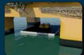
Template lowered into water with both rigs
